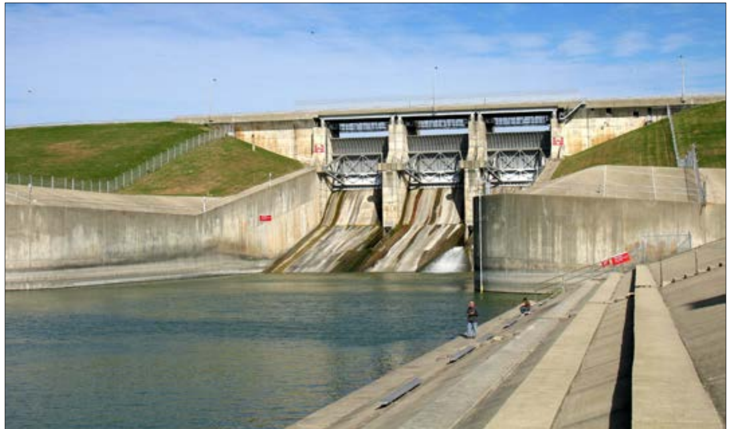
Shelbyville Dam and Spillway. Photo: https://ilickr.com/photos/yodudedan/
